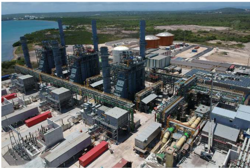
Commissioning of SJPC Power Plant
